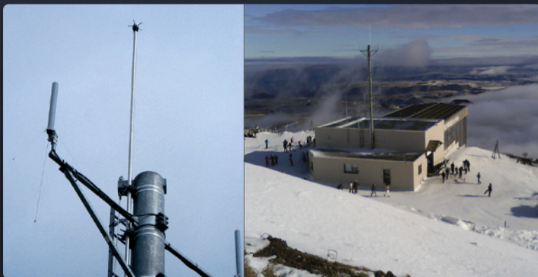
ESE air terminal in extreme climatic conditions
