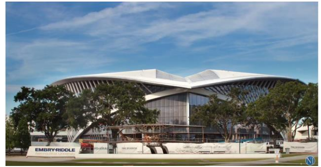
8) Building with the Lightning Protection System
