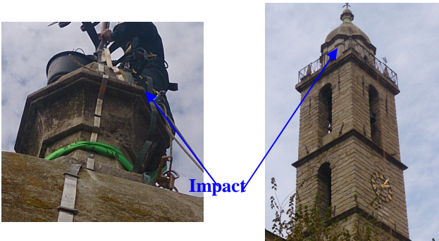
Fig. 1. church protected by a simple rod and impacted
